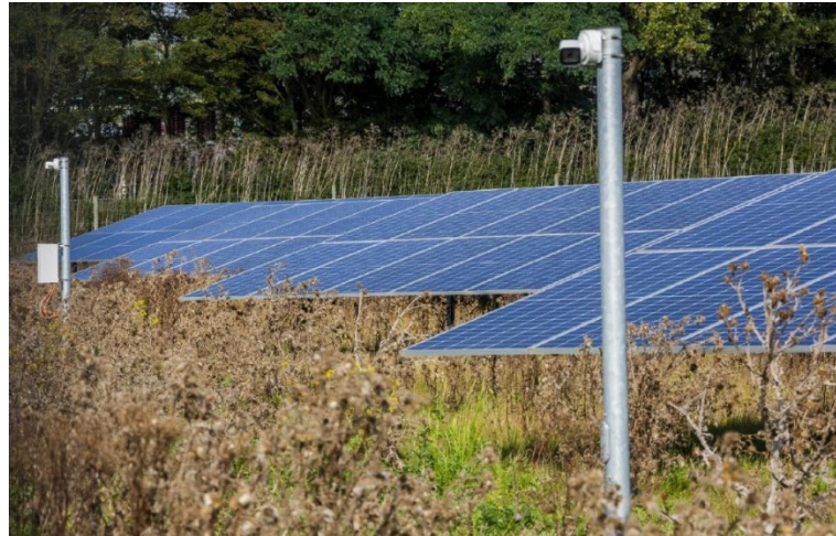
Image 9: Pole-mounted Security Camera
