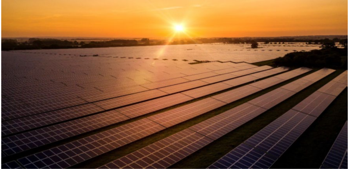
Image 2 Fixed South Facing PV Arrays
